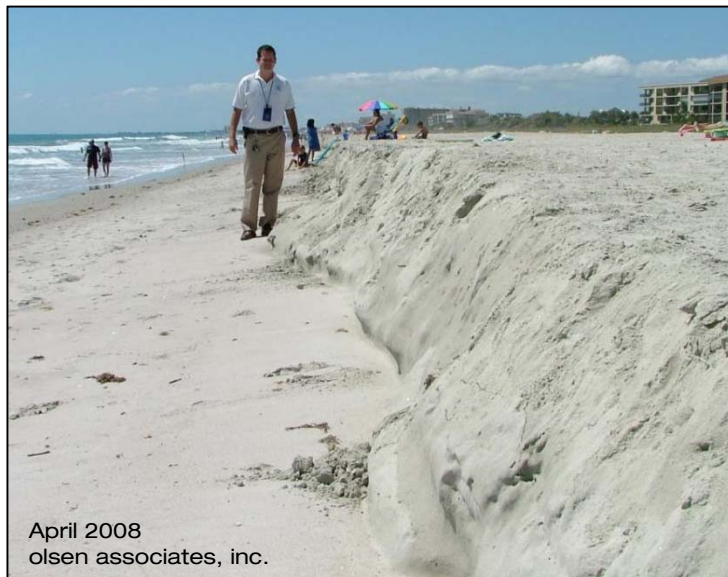
Figure 4: Escarpment along sand bypass fill area one year following Sand Bypass III in completed in 2007.
